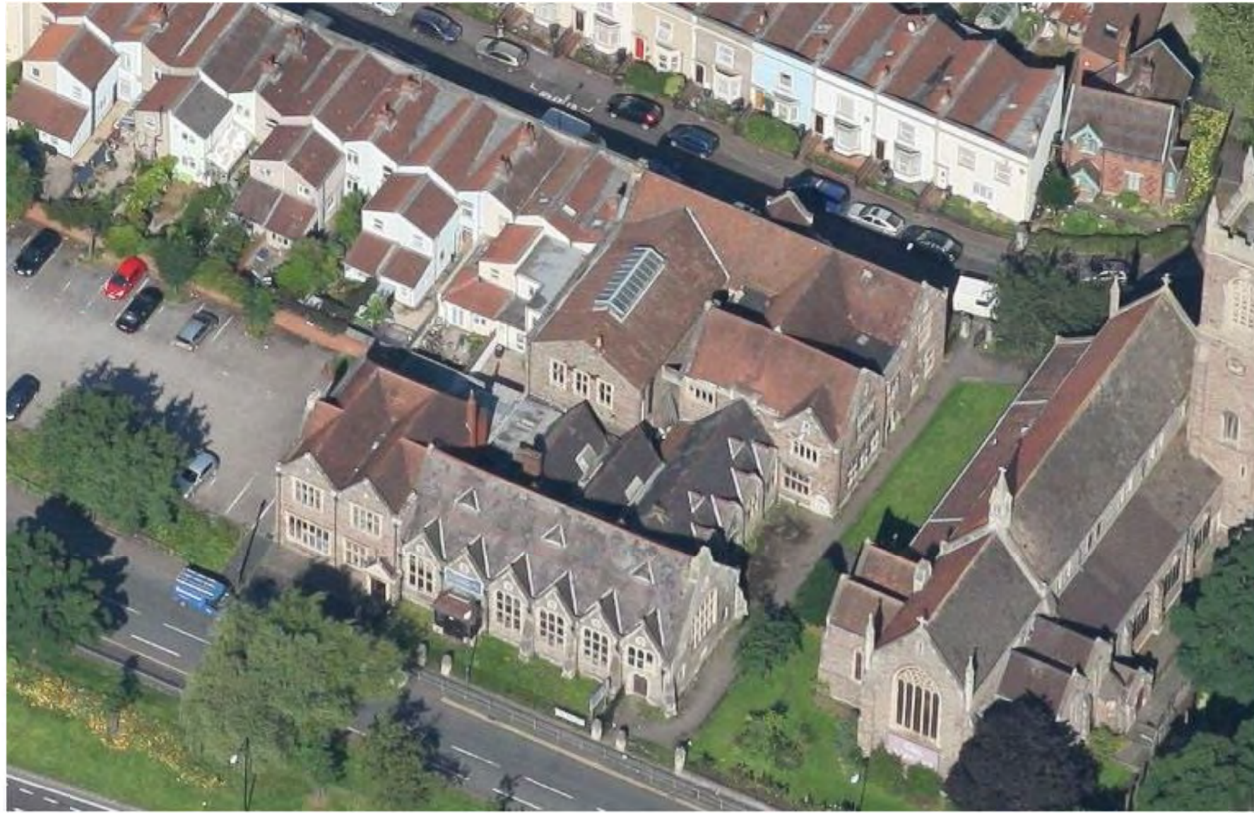
Aerial View of Existing Roofscape
